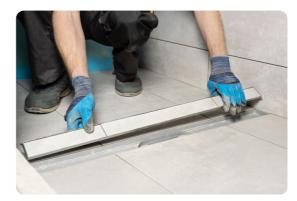
**2.** Trim the top tray 1mm shorter than the bottom tray to facilitate a smooth insertion of the top tray for a neat and snug fit.
